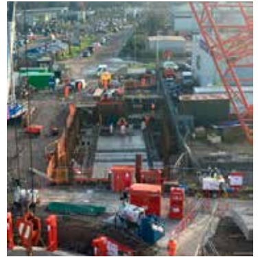
Guildford sewage treatment works is relocating to a new site.
