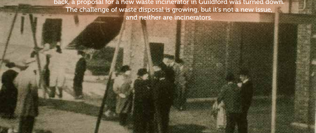
The Guildford Dust Destructor.
